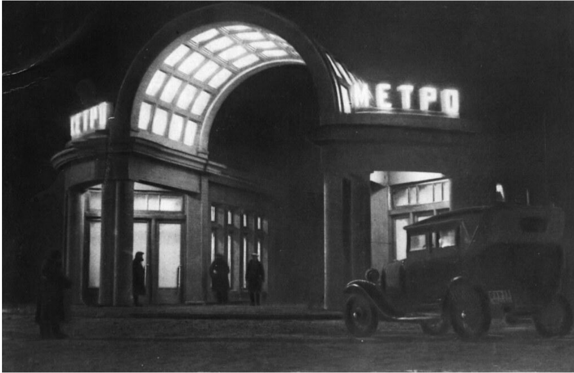
Fig. 11. Moscow Metro, "Kropotkinskaya" station, 1935
