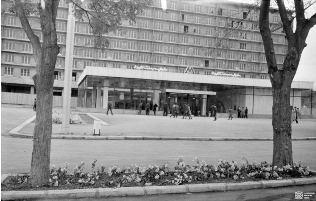
Fig.26. Metro station "26 Komisari". Central Historical Archive
