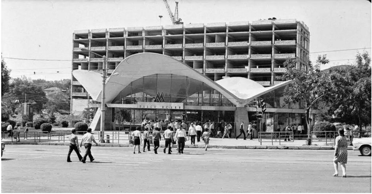
Fig.28. Metro station "Isani". Central Historical Archive
